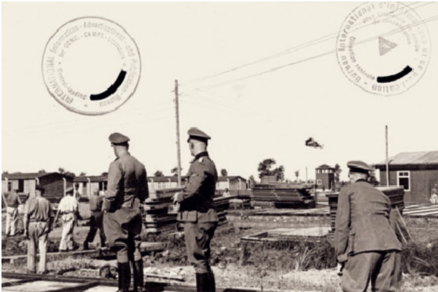
Prisoners working on the construction of the SS barracks in 1940. The prisoners' barracks can be seen in the background.
