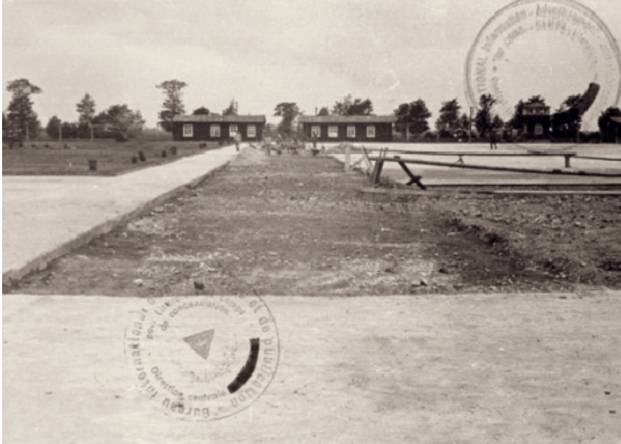
Paving work at the prisoners' barracks in 1941. The parade ground is to the right.
