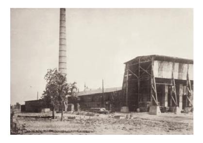
The old brickworks in Neuengamme. To the right is the provisional wet press. It was used for experimenting with different wet pressing techniques after dry pressing procedures had proven unsuitable.
